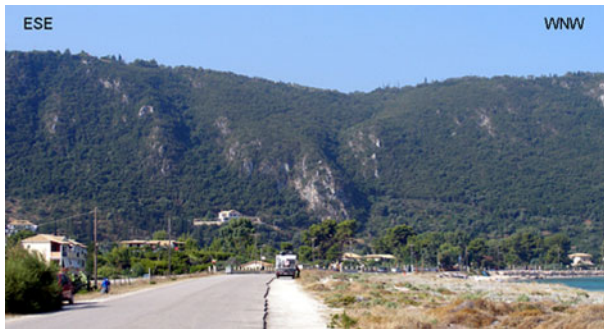
Fig. 8 View of Tsoukalades scarp, indicating gravitational instability
