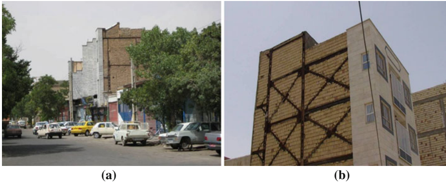
Fig. 3 Samples of Steel frame building types (Derakhshan 2009). a Simple steel frames without bracing. b Simple steel frames with bracing
