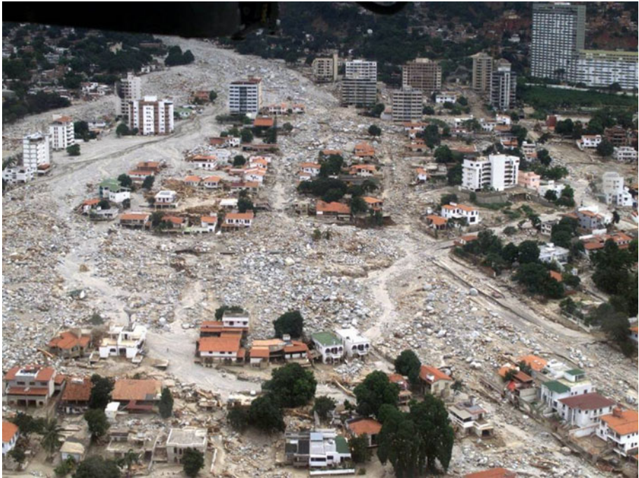
Fig. 1 Carabella, Venezuela debris flow, 1999. Damage class IV: complete destruction. The estimated I_{DF} for this event was 500. Photograph from Matthew C. Larsen, U.S. Geological Survey
