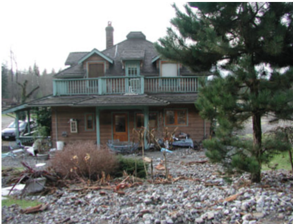
Fig. 2 Damage class I: some sedimentation for a debris flow in Hatzik Valley, southwestern B.C. The estimated I_{DF} for this event is <1 . Photograph: Matthias Jakob. November 2002
