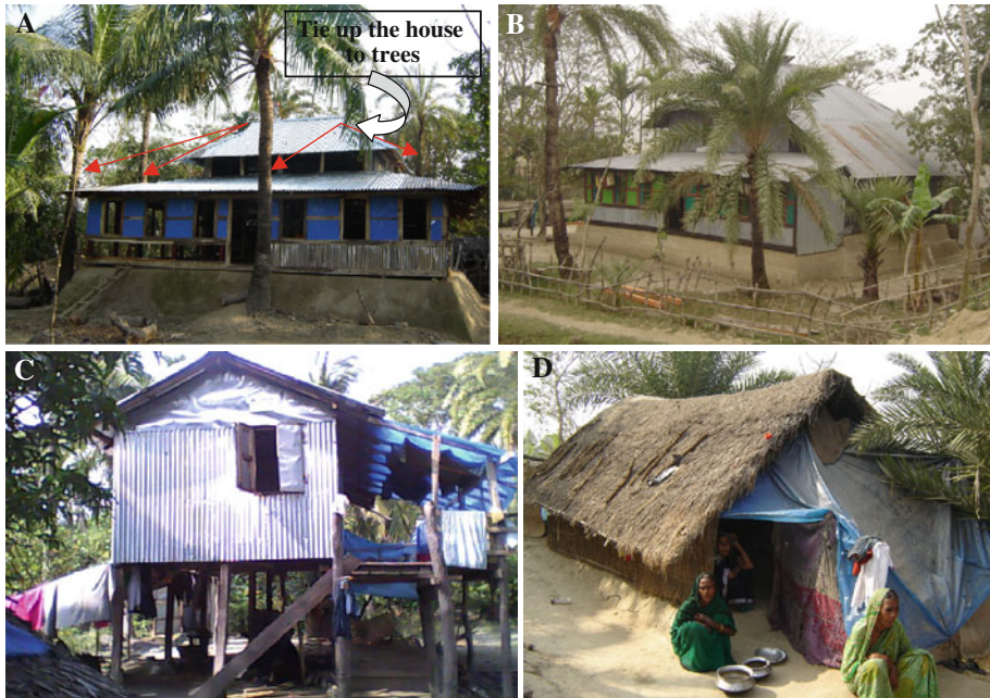
Fig. 2 a Temple shape house. b Gently sloping of the roof of the house. c Elevated house on wooden structure. d Thatch roofed house
