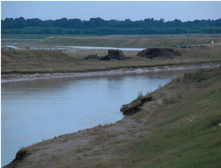
Fig. 9 Dike breached by flood in the Siret River lower watershed (Romanescu 2005)
