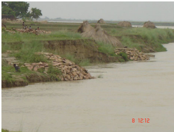
Fig. 8 River is approaching close to the settlement due to lateral erosion
