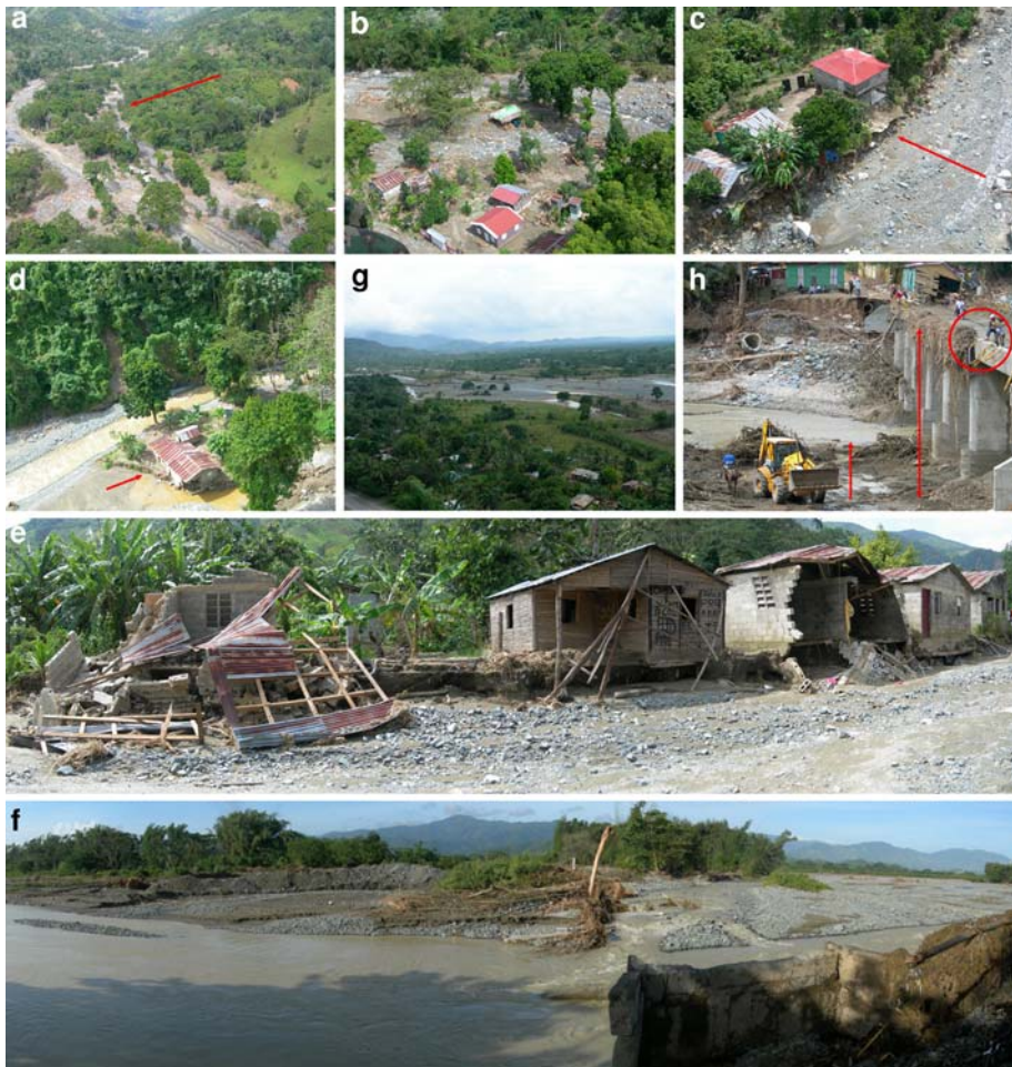
Fig. 10 Impacts of stream erosion on anthropic structures provoked by the flood during the passage of the tropical storm Noel. Note that within the surveyed fluvial reaches the damaged houses are located or on the flood plain or within the active channel (a–e); flood effects related to elevated hydrometric levels during the storm event: the collapse of the bridge on the Haina river within the Villa Altagracia municipality (f); a view from the Duarte highway, locally reached by the flood (g); evidence of the elevated hydrometric level reached by the Mahomita river within the town of Los Cacaos, San Cristóbal province (h)
