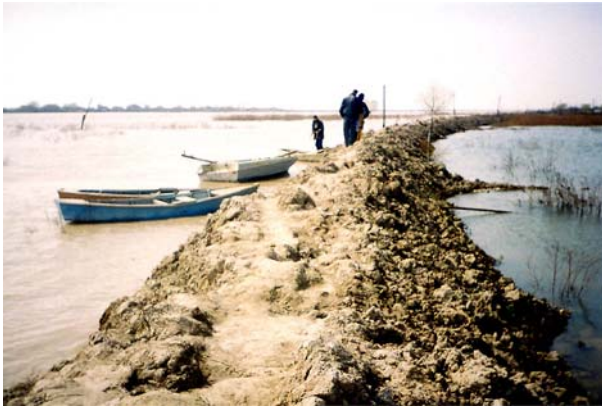
Fig. 6 Underground flooding near the outlet in 2005 (right coast)
