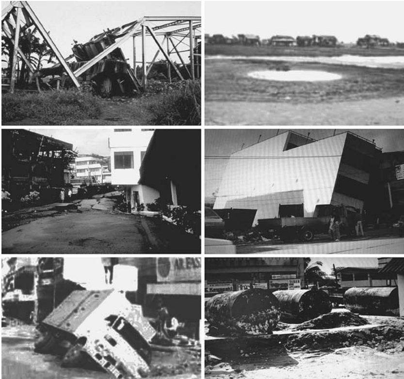
Fig. 2 Effects of liquefaction caused by the 1990 July Luzon earthquake
