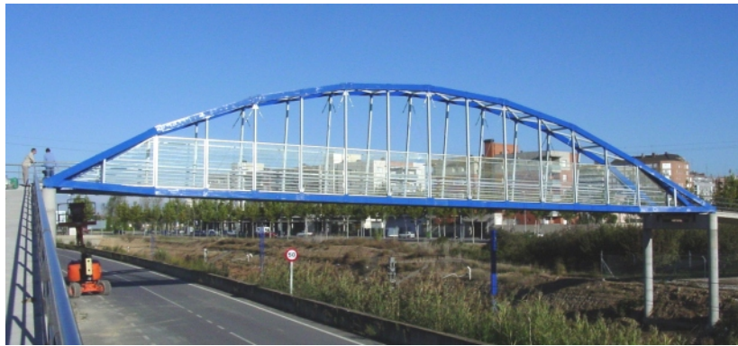
Fig. 1. GFRP footbridge in Lerida, Spain [1].
