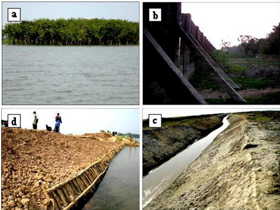
Fig. 5 (a) An established koroch plantation in the study areas (b) Traditional wave protection wall (c) Digging of canals for easy water movement and rain water harvesting (d) Construction of an embankment for the protection of agricultural field and houses from flash flood
