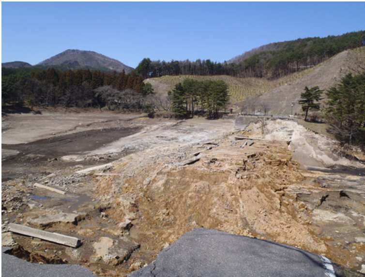
Fig. 4 Burst dam (Fujinuma reservoir)
