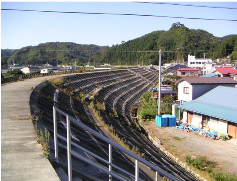
Fig. 8 Ten meter high coastal dykes in Taro, Miyako City (Before the tsunami; Ministry of Land, Infrastructure, Transport and Tourism)
