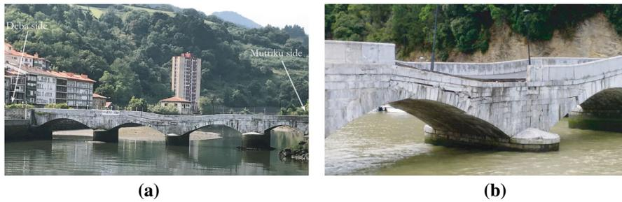
**Fig. 2** Deba bridge failure under pier settlement induced by pile shipworm infestation: **a** general view; **b** second pier
