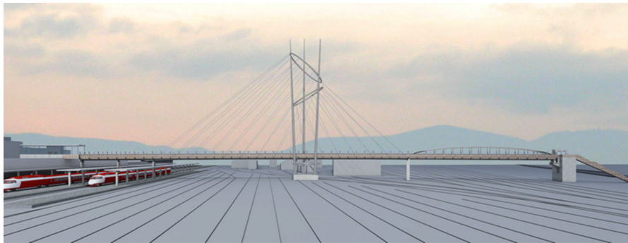
Fig. 1 View of the “Umbria Gateway” cable-stayed footbridge
