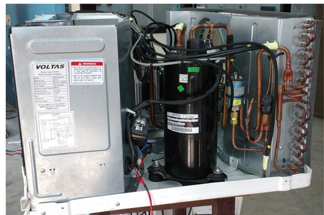
Fig. 4 Photographic view of the test room air conditioner
