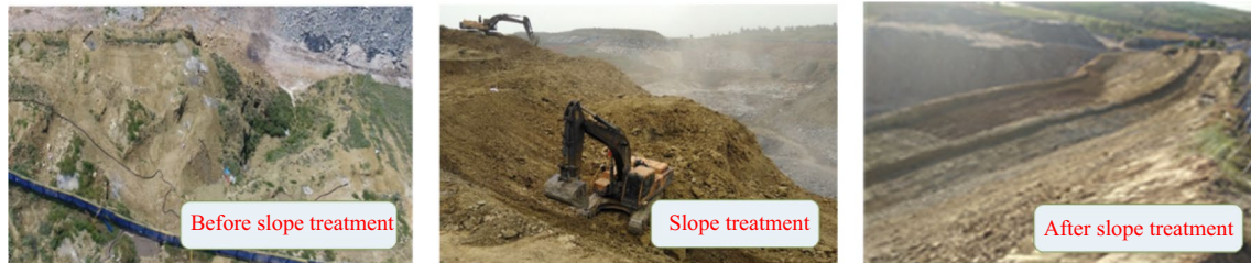
Fig. 11 Slope treatment to prevent air leakage
