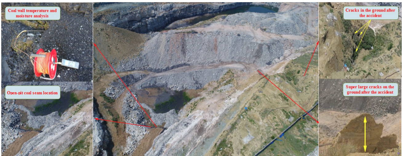
Fig. 4 Ground condition after accident
