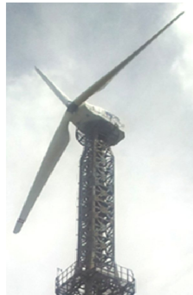
Fig. 5 INER-P150II wind turbine
