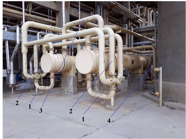
Fig. 1 Real shell and tube cooling heat exchangers of the RFCC gasoline product that have been modeled. (1) Inlet cooling water to tubes, (2) outlet cooling water from tubes, (3) inlet gasoline product to shell, (4) outlet gasoline product from shell
