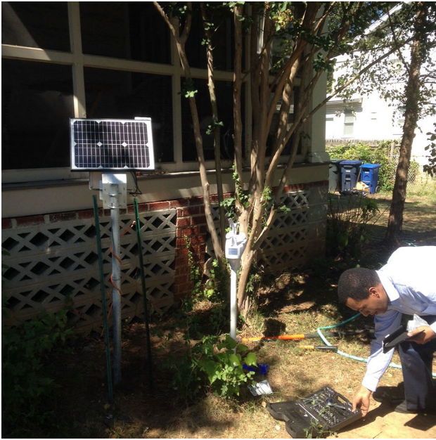
Fig. 6 A monitoring system installed in Washington D.C
