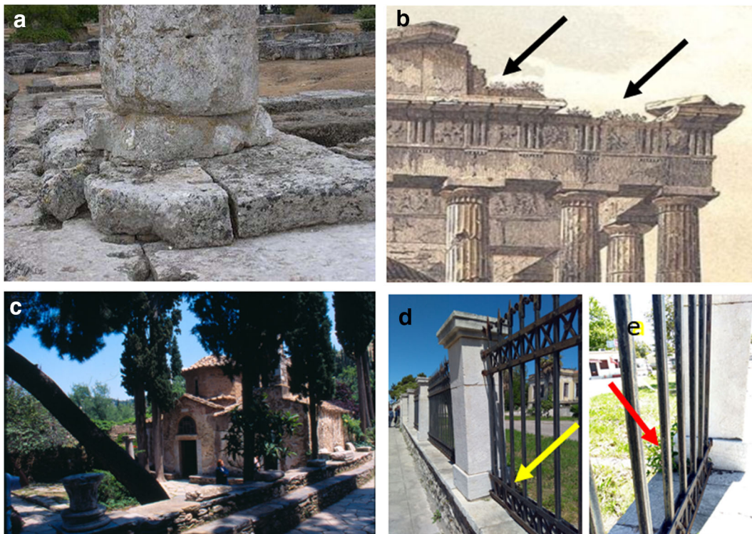
Fig. 10 Effects of plants in the structural stability of ancient monuments. a Poor condition of the base of one of the three surviving columns of the Nemea Temple, assigned to root action before the excavation of the lower part of the column (Hill 1966) or to unsuccessful efforts at undermining the column (Miller 1986) (after Makris and Psychogios 2004 and Miller 1986). b Plants in the superstructure of the east façade of Hephaisteion Temple in
