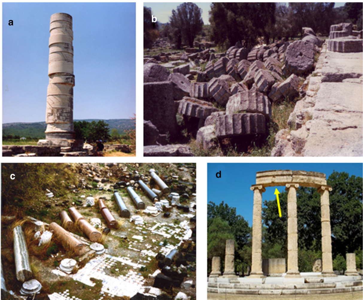
Fig. 2 Damage and repairs in ancient columns. a Offsets in drums in the Hera Temple, Samos Island, Greece. b Temple of Zeus, Olympia, drums of columns collapsed in a domino-type pattern. This collapse in Later Antiquity postdates a repair of the temple probably in the second century BC. c A well-known case of oriented collapse of columns in the internal part of a basilica at
