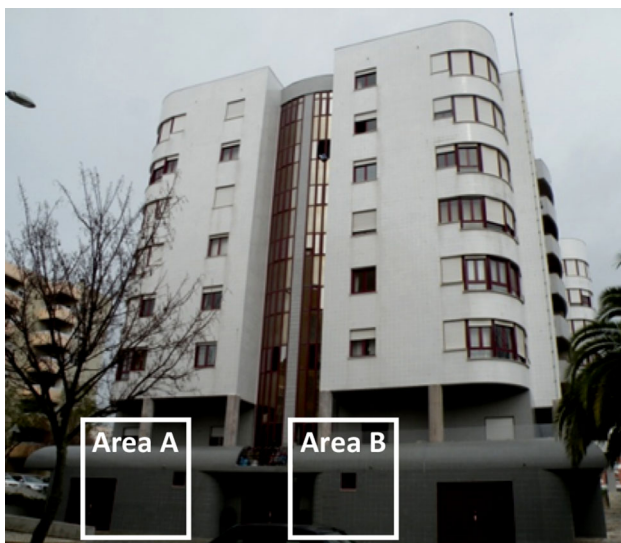
Fig. 10 Photograph of building B-11's south facade and areas of interest
