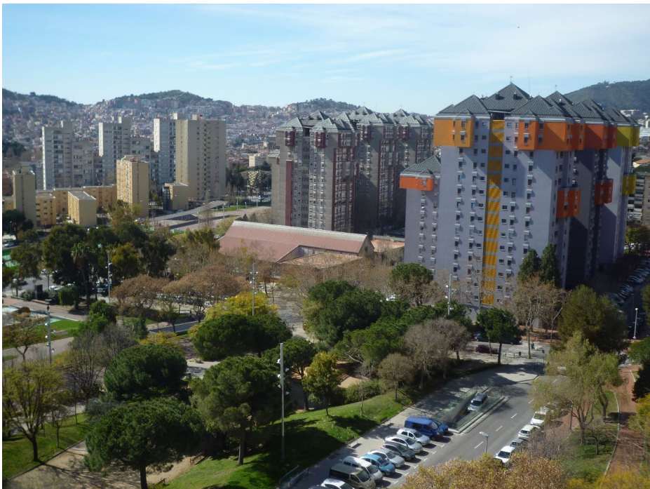
Fig. 4 Refurbishment of the towers of Canyelles. Sources: the authors March 2019
