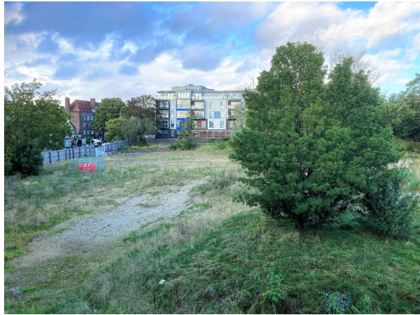
Fig. 9 Empty site (foreground), old social housing block (left background) and new housing block (centre background) at Clapham Park south, 2021 Photo: Paul Watt
