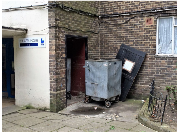
Fig. 3 Bin area (with broken-off door) outside social housing block at Clapham Park west, 2016 Photo: Paul Watt
