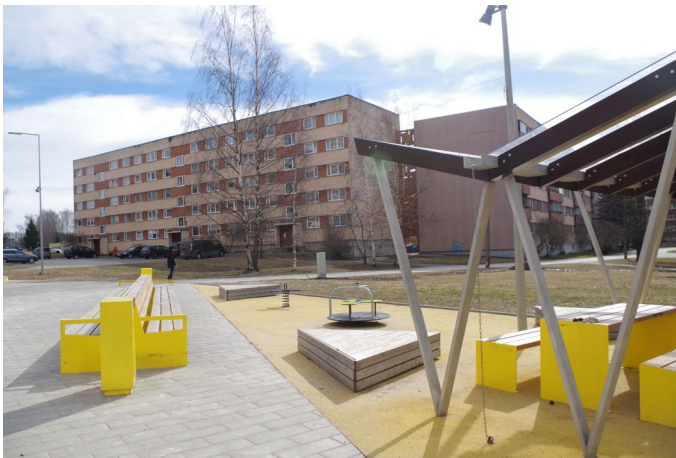
Fig. 6 The finished public space improvement project in 2017. Photo: J. Pirrus
