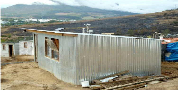
Fig. 1 Design of the improved shack in Enkanini-Stellenbosch, South Africa. Source: The iShack Project was pioneered by the Sustainability Institute of Stellenbosch University, 2016
