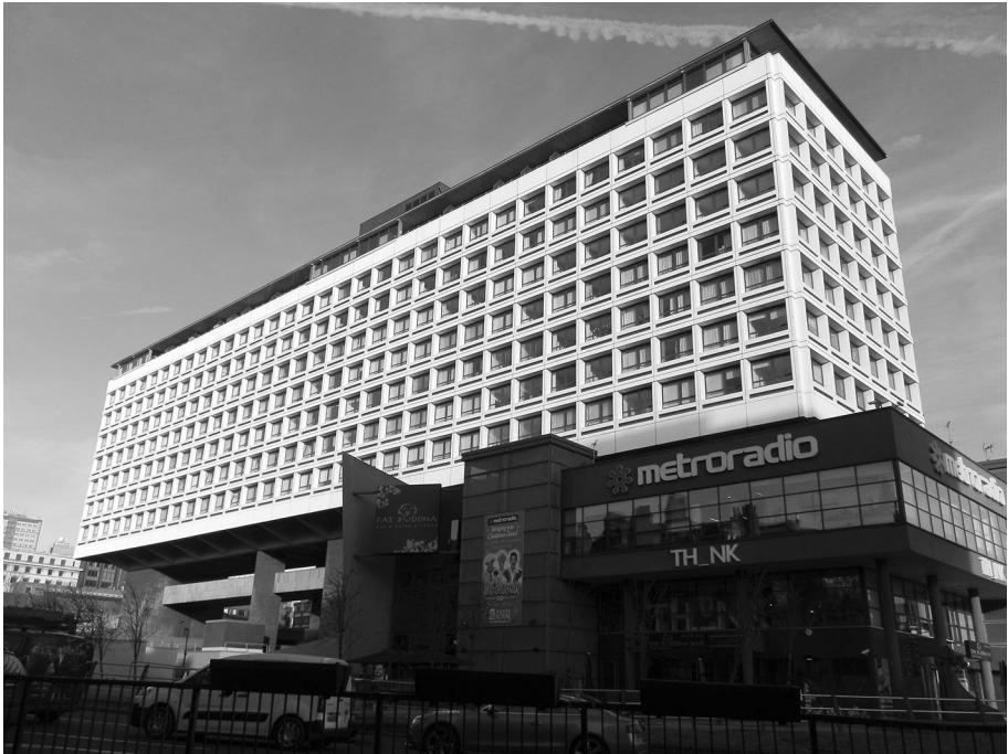
Fig. 11 55 Degrees North (former Swan House roundabout) (Photo: M. Barke)
