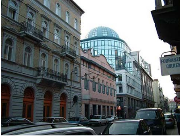
Fig. 3 Suba Office Centre among recently renovated residential buildings in Inner-Terézváros. Photo: Z. Földi, September 2004
