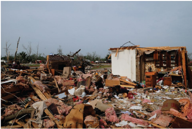
Fig. 1 Severe damage caused by a tornado. A priori information about the environment would be out of date due to the large amount of debris [7]
