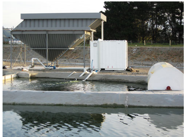
Fig. 6 Photograph of the Christchurch demonstration algal harvester
