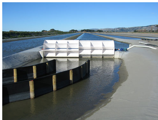
Fig. 4 Photograph of the Christchurch demonstration HRAP paddlewheel
