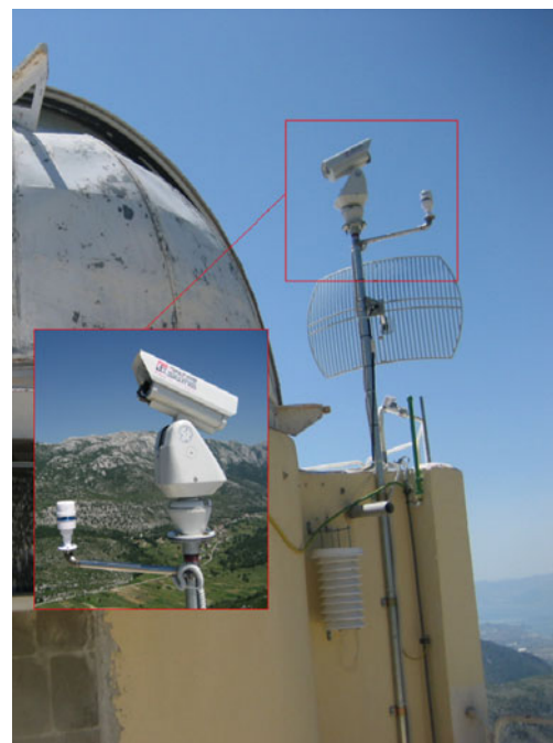
Fig. 7 Monitoring station mounted on existing infrastructure (astronomical observatory)
