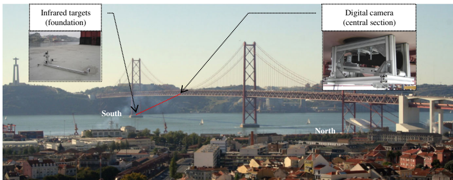
Fig. 2 25th of April Bridge showing the location of the optical displacement measurement system
