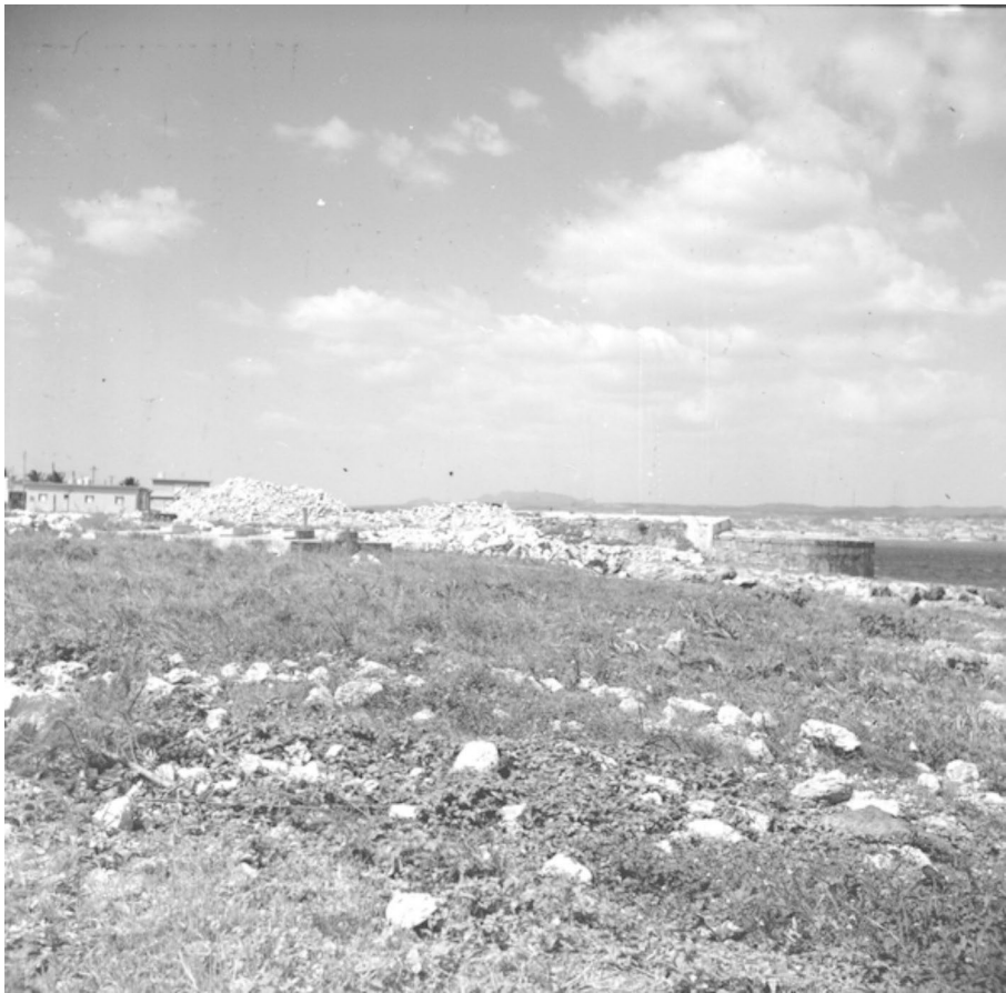
Fig. 11 Photographs dating from 1962 showing piles of debris, and part of the preserved semicircular battery.
