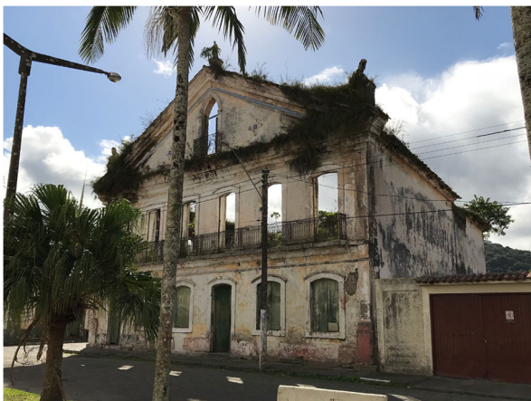
Fig. 1. Current Situation of the Building. Credit: Wagner Magalhães – July 2018
