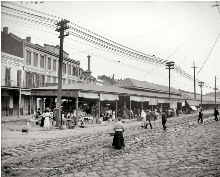
Fig. 7 1910 photo of market buildings (Library of Congress)
