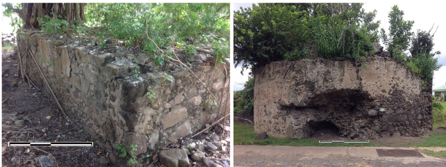
Fig. 4 Left: detail of large indigo vat at Park (note irregular coursing of masonry; this feature was largely destroyed during development in 2015); and right large lime kiln structure at Pagets Farm. Scales: 1 m
