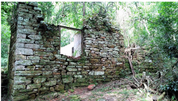
Fig. 1 Lateral wall of Structure I. Notice the use of almost uncut stone and the modern machine-made window
