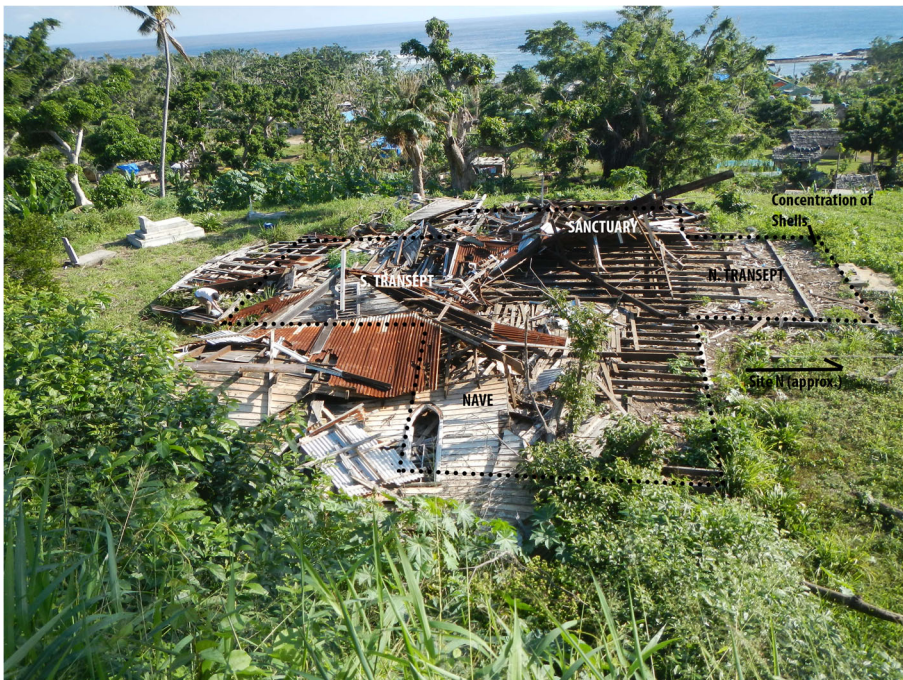
Fig. 1 The 1912 Lenakel Church after Cyclone Pam. The dotted line represents the approximate outline of the church footings. Note how the structure was blown to the south by the strong northerly winds of the cyclone, which reached 280 km/hr
