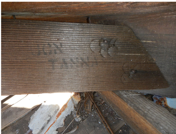
Fig. 2 Previously unseen dispatch marks, such as this were accessible after the building’s destruction. Note also the hammer marks where the nails were driven into this roof rafter
