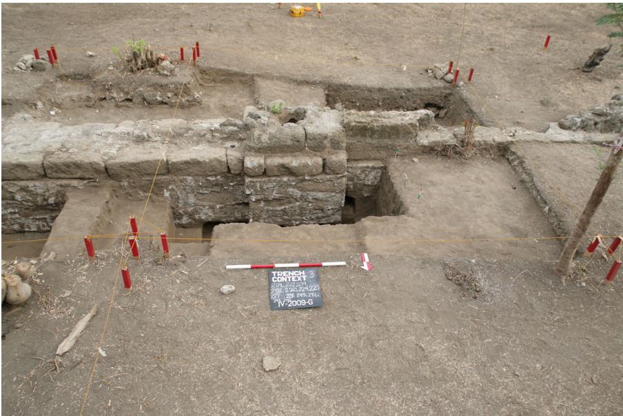
Fig. 19 The south wall of Structure B showing the difference in wall thickness, materials used, and foundation depths of the west side and east side
