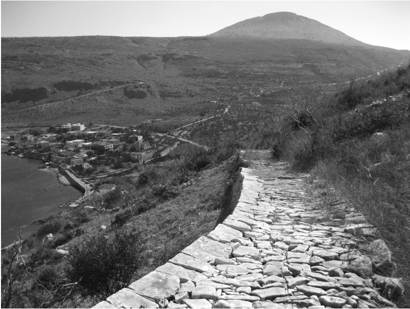
Fig. 5 Kalderimi leading from Areopoli to Kelepha, looking northeast
