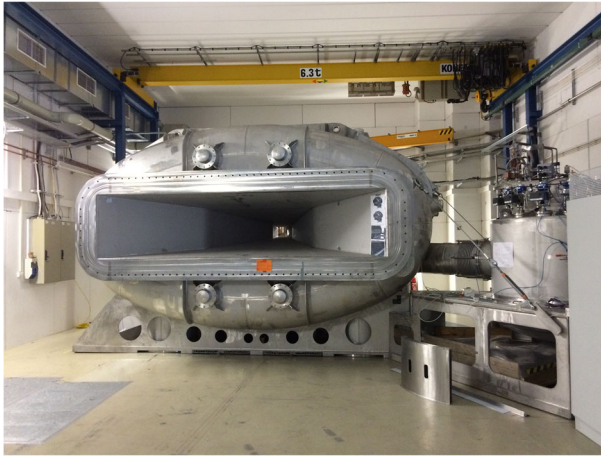
Fig. 2 GLAD magnet shortly after its move into Cave C of GSI. It will stay at this position until the final move to the high-energy cave of the FAIR facility
