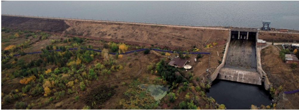
Fig. 1. Photo of the structures of the Verkhneural'sk hydraulic unit.
