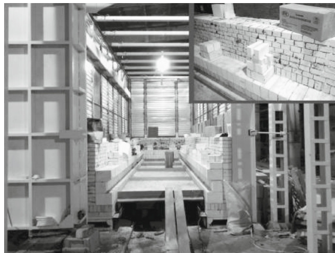
Fig. 3. Lining of the high-temperature furnace at Rechitskii farfrovyy zavod, JSC.
