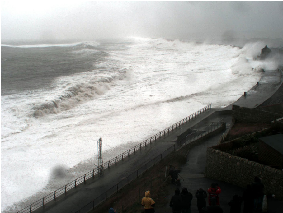
Fig. 3 Example of coastal defence overtopping at Chesil Beach, UK, caused by extreme swash events exceeding 10 m (see Poate et al. 2016) during Petra storm on February 5, 2014 (credits: Tim Poate)
