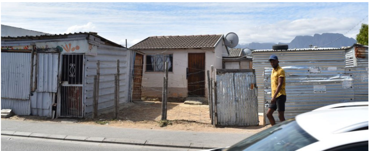
Fig. 12 Informal extensions using temporary materials. (Author's own)
