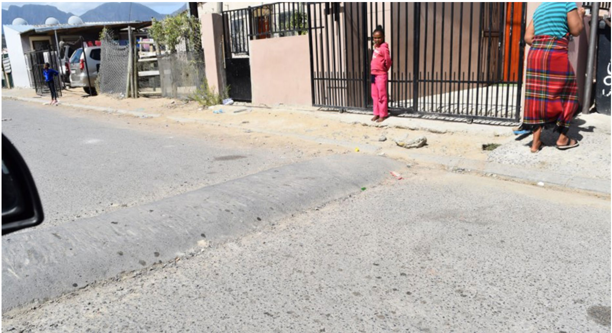
Fig. 13 Informal traffic calming measures erected by the community. (Author’s own)
