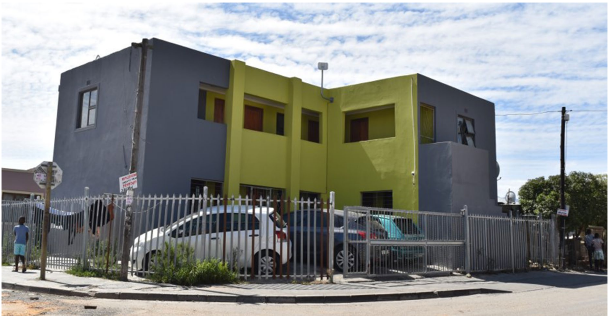
Fig. 5 A multi-level apartment redevelopment in Zola. (Author's own)
