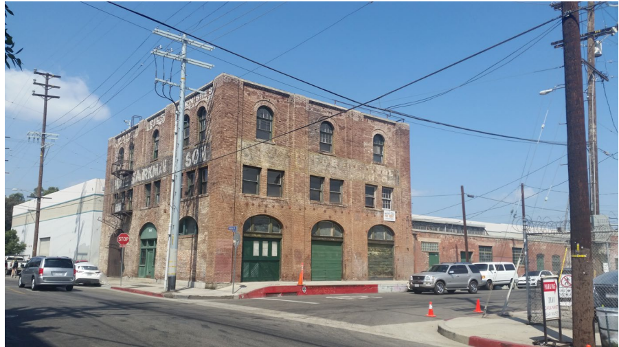
Fig. 1 The Nate Starkman Building in 2016
