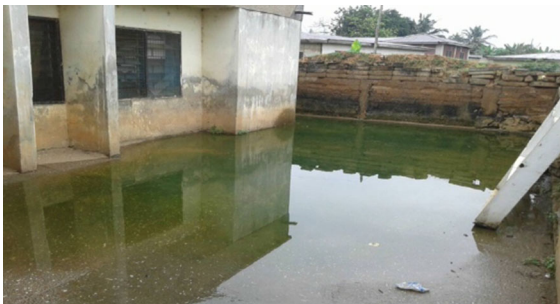
Fig. 3 Residential facility within a wetland, Dichemso
