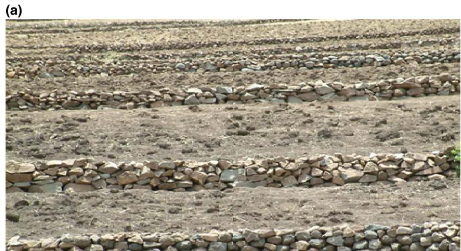
Fig. 3 a Stone bund constructed on sloping area of Debre Tsyon kebele. b Terraces constructed on sloping area of Debre Tsyon kebele
