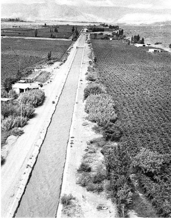
Fig. 2 Channels of the artificial irrigation network
