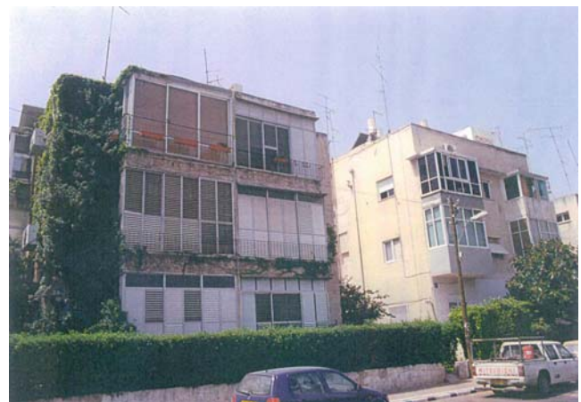
Figure 8. Baret: nearby old buildings.
