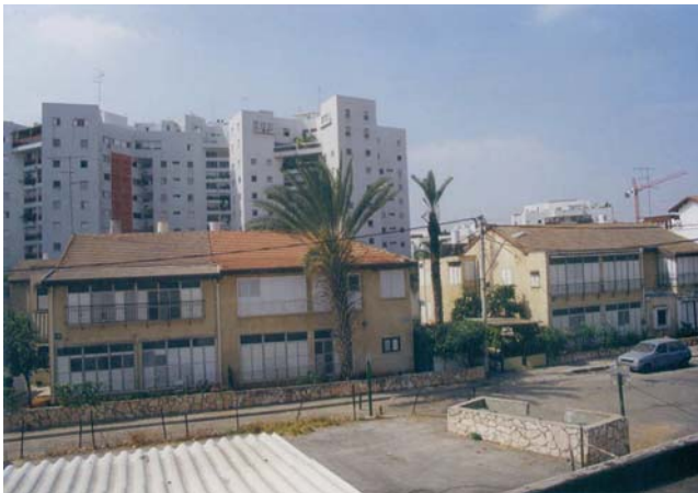
Figure 2. Yahalom: old buildings in foreground, some refurbished, new buildings in background.
