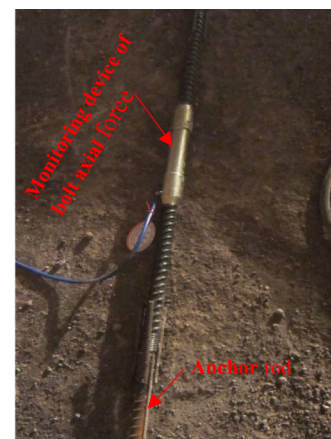
(b) Monitoring device installation
